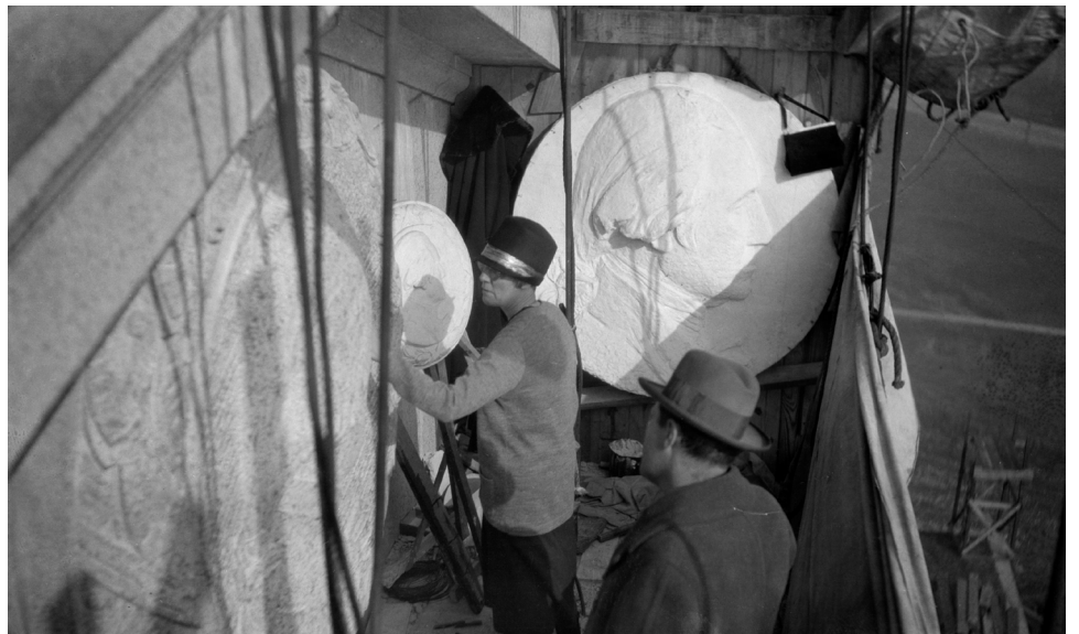
TOP: The fully-restored pediment. MIDDLE LEFT: The uncarved granite. MIDDLE RIGHT: In 1927, the medallion of George Washington's profile was carved on site from a box scaffold. BOTTOM: Gail Sherman Corbett puts the finishing touches on the Portico's medallion, with her original plaster maquette and a larger plaster model on hand for direct comparison.
