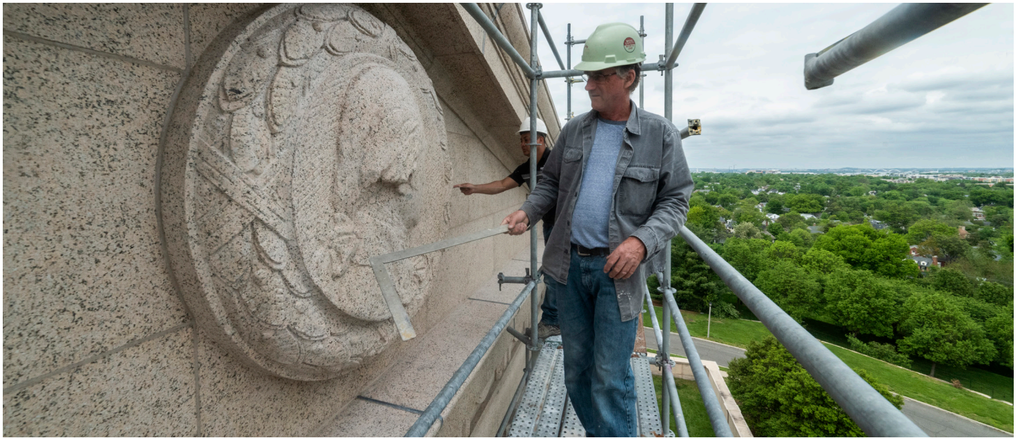
Paul Keegan of Hibernia Masonry prepares to measure the medallion after cleaning. It is 78 inches (6½ feet) in diameter. It is carved from a single block of granite.
